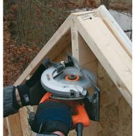
Create a pocket for the ridge. At the top of the center stud, I finish the plunge cut that I started before I assembled the wall. Once the cut is complete, I remove the two screws holding the top plate to the center stud, remove the piece, and drop the ridge board into place.
