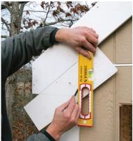
Use a level to scribe the rake return quickly. I tack a short piece of trim in place along the rake, then scribe the vertical and horizontal cuts.
