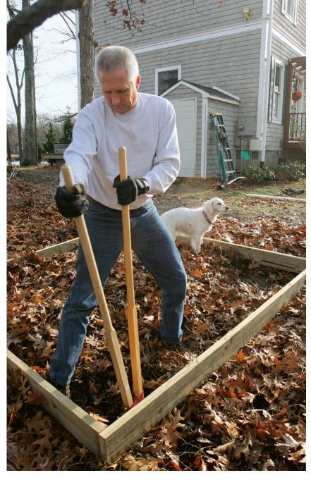
**PVC piers are easy to level.** Fit all four PVC piers in their bases, and set them in their holes. After cutting the first one a few inches above grade, I level across to mark the cutlines on the other three.
