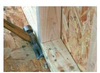
Fine-tune the wall placement with the holding nail. Before I build the wall, I snap a layout line 3½ in. in from the edge of the floor and toenail the bottom plate to the inside. When I stand the wall, the nails keep the wall from sliding off the floor. Once the wall is up, I can move the wall back to the line by bending the nail with a hammer.
