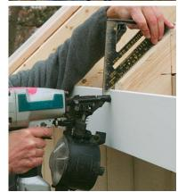
Locate the fascia with a straightedge. I hold my Speed Square on top of the rafter and butt the top edge of the fascia against the square before nailing it fast. This ensures that the roof sheathing is not pushed up where it meets the fascia.
