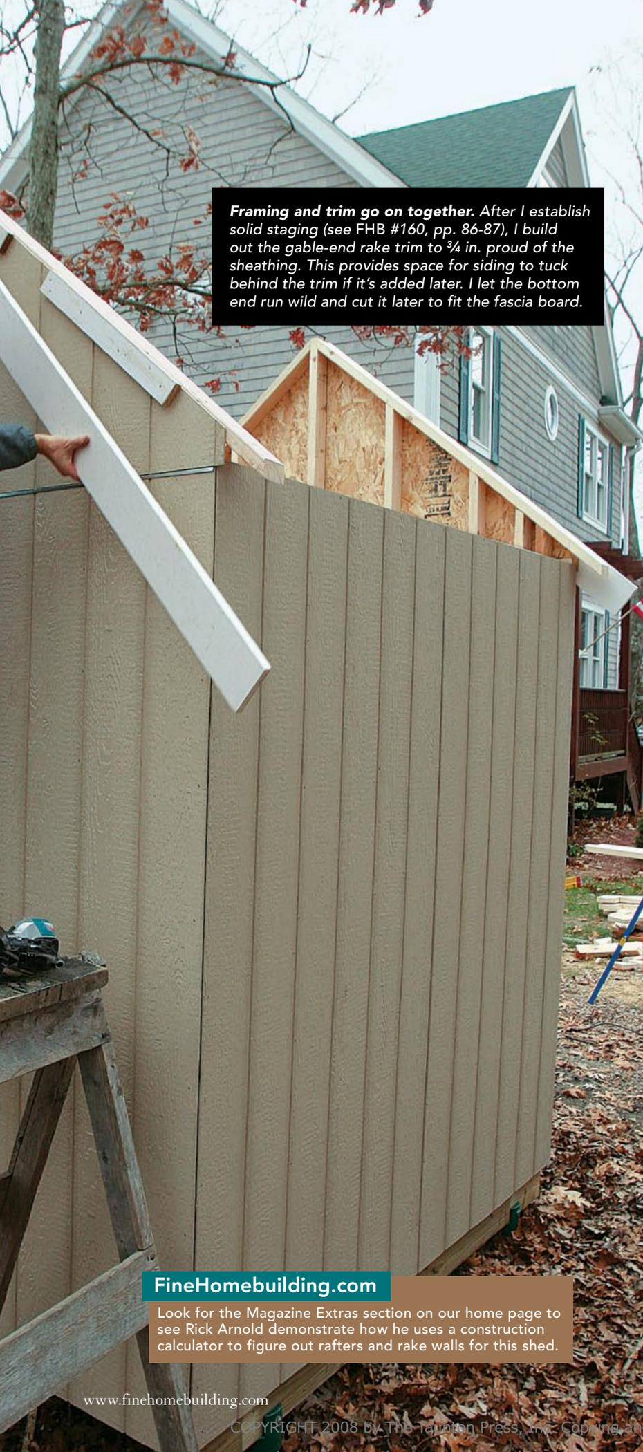
**Framing and trim go on together.** After I establish solid staging (see FHB #160, pp. 86-87), I build out the gable-end rake trim to 3/4 in. proud of the sheathing. This provides space for siding to tuck behind the trim if it's added later. I let the bottom end run wild and cut it later to fit the fascia board.
