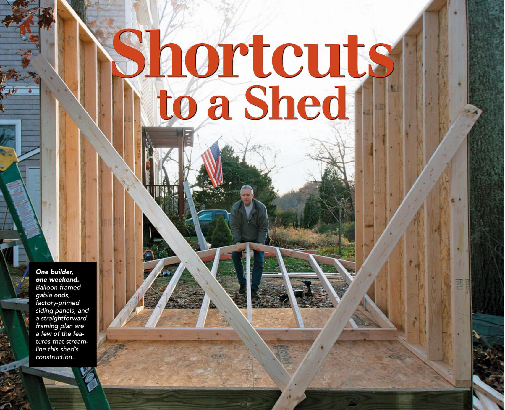
**One builder, one weekend.** Balloon-framed gable ends, factory-primed siding panels, and a straightforward framing plan are a few of the features that streamline this shed's construction.
