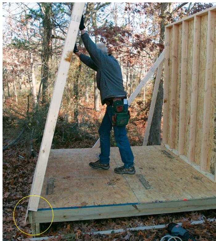
**Let the walls lean out and the siding hang down.** Once the wall is up, I brace it leaning out so that I can easily build and stand the gable walls on the floor deck. The 7-ft.-5-in. wall height allows the siding to hang down past the floor framing and act as a drip edge.
