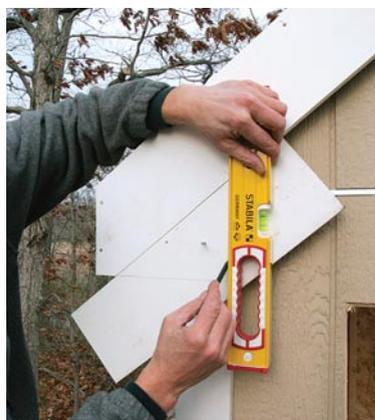
**Use a level to scribe the rake return quickly.** I tack a short piece of trim in place along the rake, then scribe the vertical and horizontal cuts.
