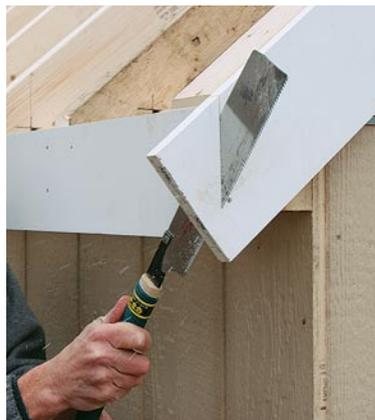
**Cut the rake trim flush with the fascia.** Once I've secured the rake trim to the fascia with a couple of trim nails, I use the edge of the fascia to guide the plumb cut on the rake trim. Then I make a horizontal cut even with the bottom of the fascia.
