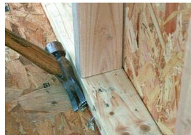
**Fine-tune the wall placement with the holding nail.** Before I build the wall, I snap a layout line 3½ in. in from the edge of the floor and toenail the bottom plate to the inside. When I stand the wall, the nails keep the wall from sliding off the floor. Once the wall is up, I can move the wall back to the line by bending the nail with a hammer.
