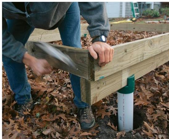
**Beams eliminate the need for joist hangers.** I let the side rim joists overlap each double 2x6 beam. This creates a ledge inside the rim that supports all the joists. I toenail the rim and joists to the beam for a solid connection.
