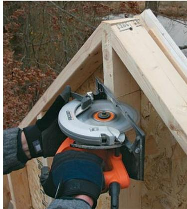
**Create a pocket for the ridge.** At the top of the center stud, I finish the plunge cut that I started before I assembled the wall. Once the cut is complete, I remove the two screws holding the top plate to the center stud, remove the piece, and drop the ridge board into place.
