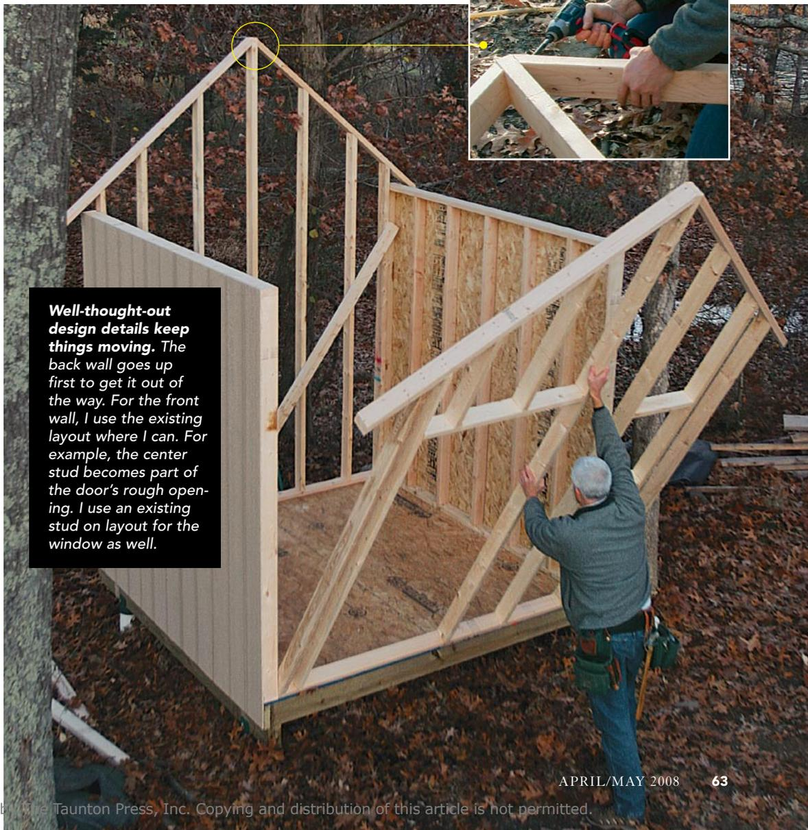
**Well-thought-out design details keep things moving.** The back wall goes up first to get it out of the way. For the front wall, I use the existing layout where I can. For example, the center stud becomes part of the door's rough opening. I use an existing stud on layout for the window as well.
