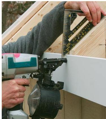
**Locate the fascia with a straightedge.** I hold my Speed Square on top of the rafter and butt the top edge of the fascia against the square before nailing it fast. This ensures that the roof sheathing is not pushed up where it meets the fascia.
