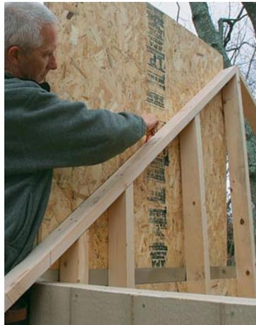
**Mark but don't measure the gable end.** I could work out this rake cut on the calculator, but in this instance, it's more efficient to hold the panel in place to mark the cutline. If I'm lucky, I can cut one side and have a big enough piece left for the other side.
