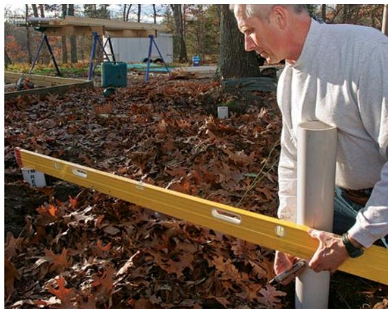
**PVC piers are easy to level.** Fit all four PVC piers in their bases, and set them in their holes. After cutting the first one a few inches above grade, I level across to mark the cutlines on the other three.
